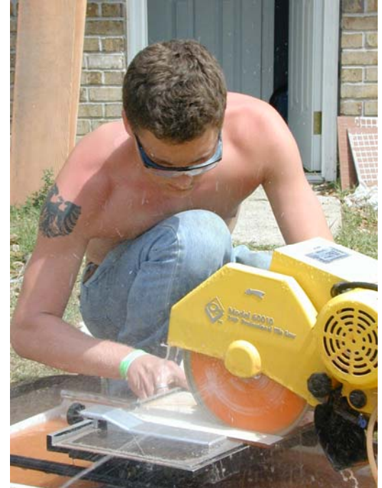
Adam cuts ceramic tiles for flooring.
